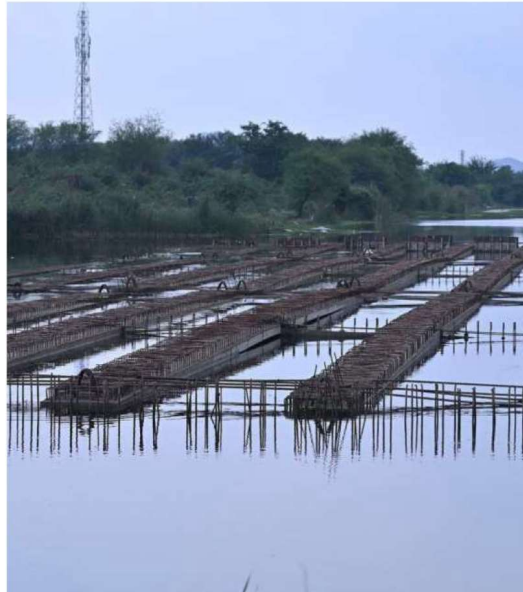
In progress: Ongoing construction of the bridge at Amaravathi, Andhra Pradesh on June 10. RAO G.N.
